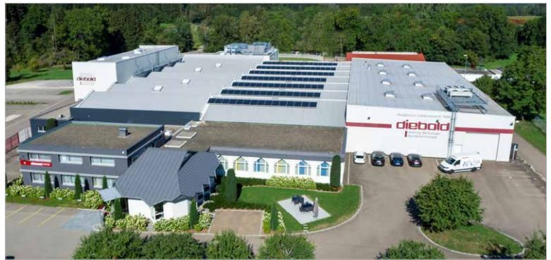
Firma Diebold "Die klimaneutrale Fabrik"
